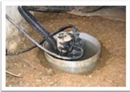
Basement/Crawlspace Sump Pumps
