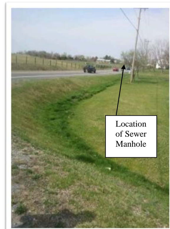
“Big Picture” of the ditch line and nearest connection.
