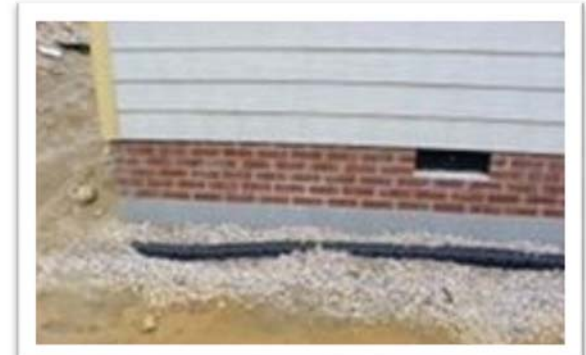
Foundation/Footing Drains
