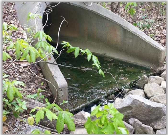
Figure 5: Example Photo showing algae growth
