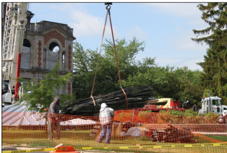
Metal braces from the old skylight
